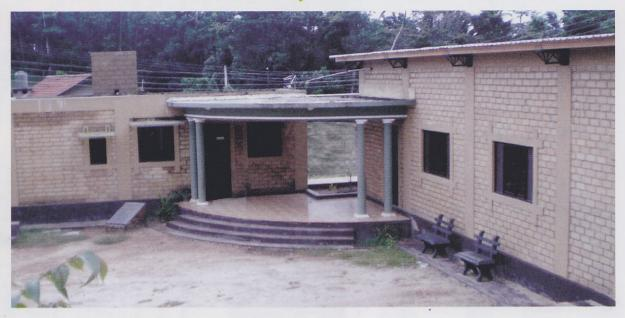
ud bricks have been used since ancient times but is still a viable, modern building material. Sun-dried mud bricks are a zero-carbon product, when it is not stabilised with cement or lime, making it one of the few eco-friendly products available in the construction industry.
